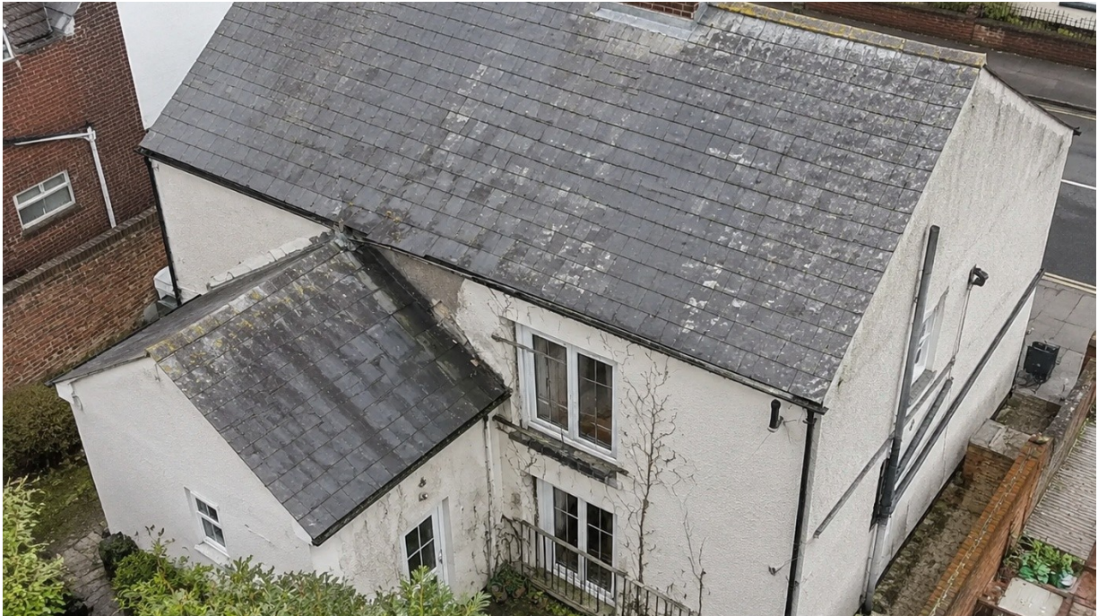
IMG-0001 • Rear oblique property overview
