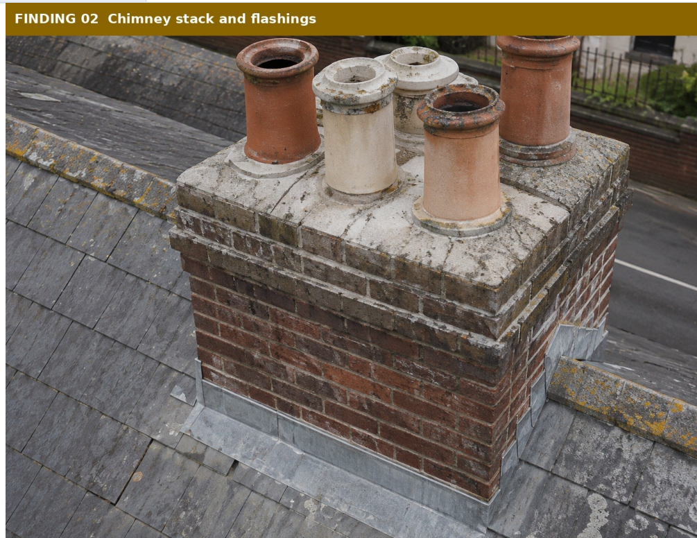
IMG-0005 • Chimney detail
