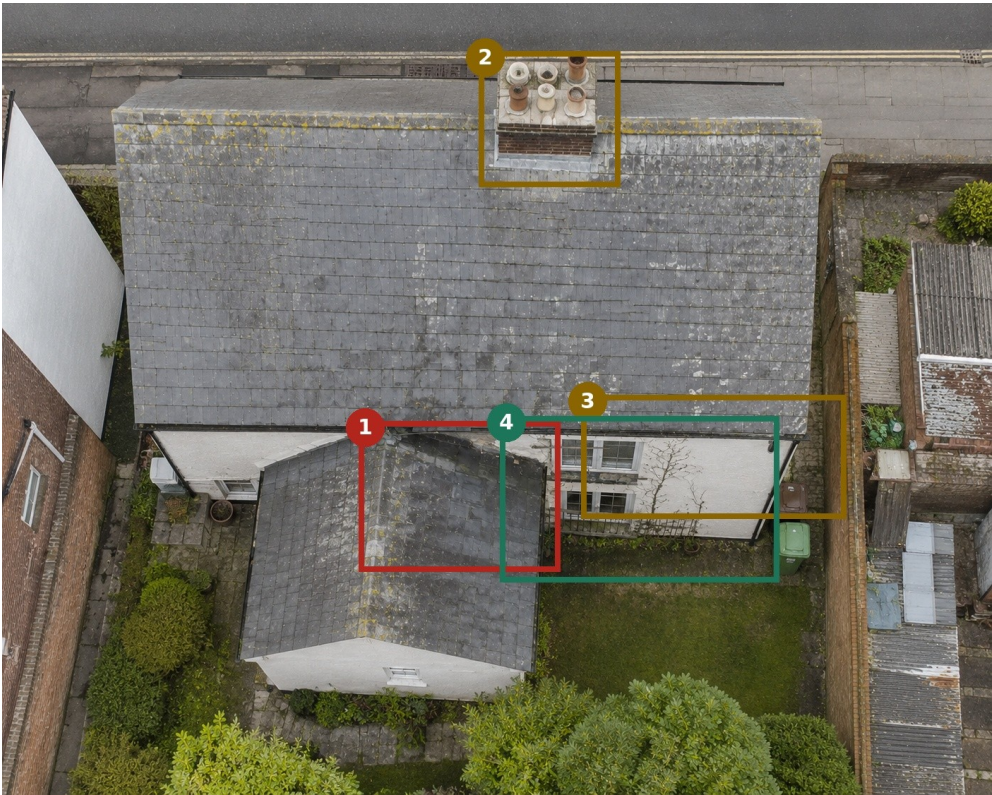
IMG-0002 • Near-vertical roof plan with finding locations
