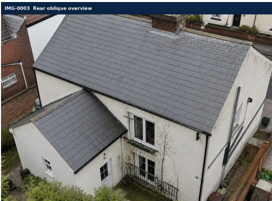
IMG-0003 • Rear slope
